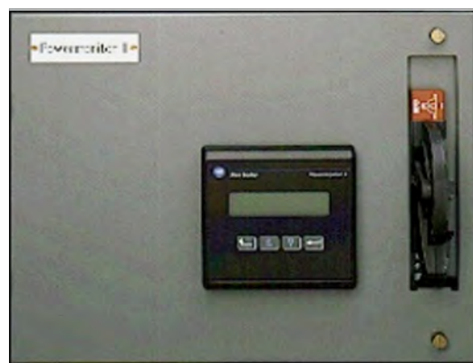
Powermonitor II Metering Unit
