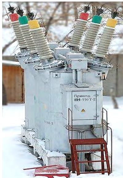
Figure 3.29: Oil circuit breaker MKP-110 (110 kV) on traction substation 110 kV 50 Hz/3.3 kV DC of railway, Toliatti city, Russia. By: Vivan.
